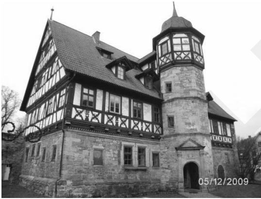
Figure 2. Damenstift Wasungen road side.
