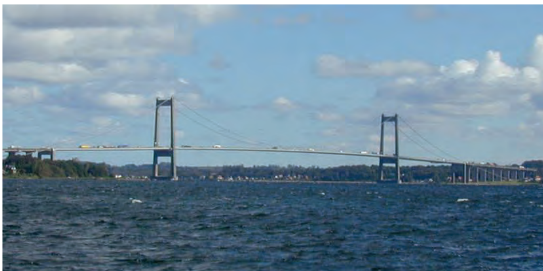
Figure 2. The layout of Lillebaelt Bridge (source: http://static.panoramio.com/ )
