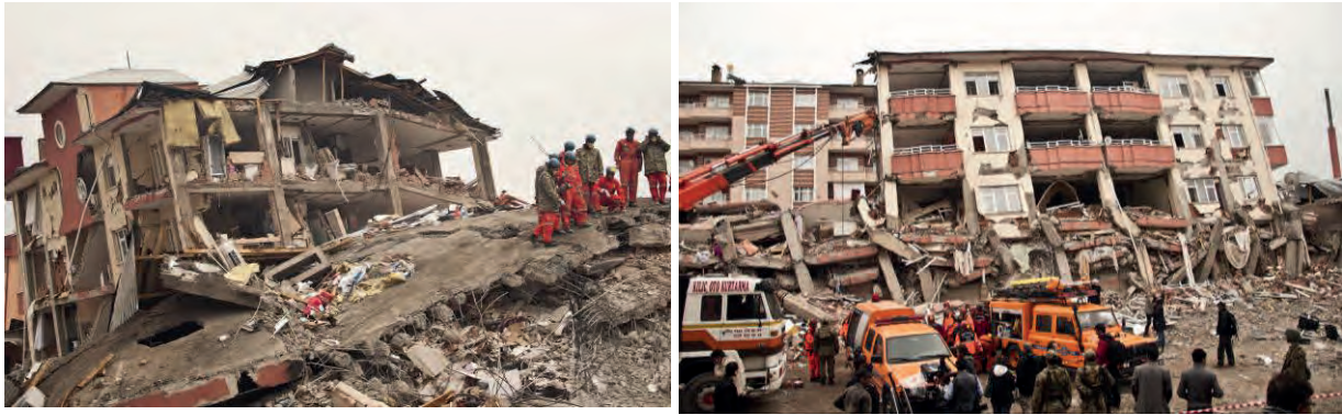
Figure 3. Damages of buildings after the Van earthquake, 2011
