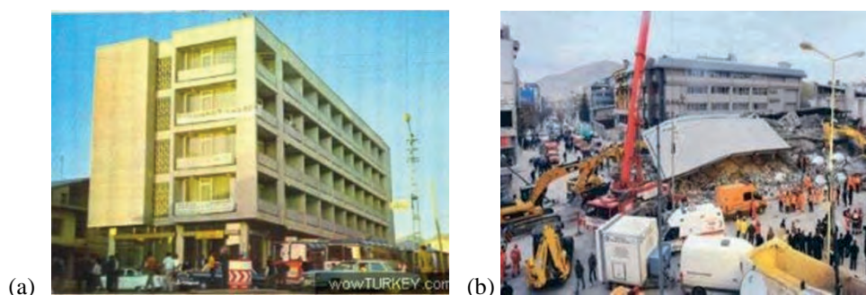
Figure 11. Building in Turkey: (a) After the main-shock, October 2011 and (b) collapsed building due to the after-shock, November 2011
