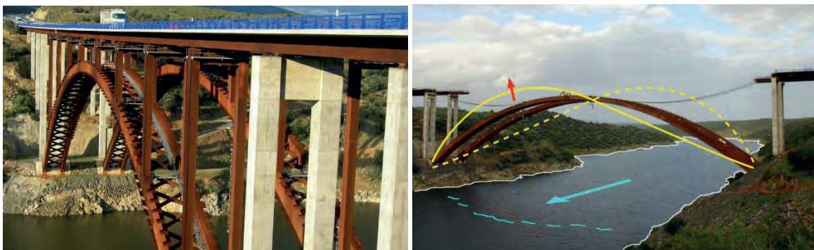
Figure 1. General View of Alconétar Bridge (left), vortex-induced motion of the bridge (right) [3, 4]
