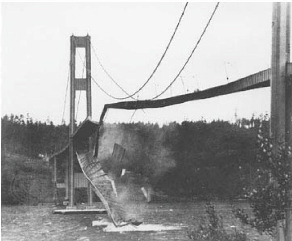
Figure 2.2: Tacoma Narrows Bridge collapse (picture courtesy of Wikimedia Commons contributors, commons.wikimedia.org).
